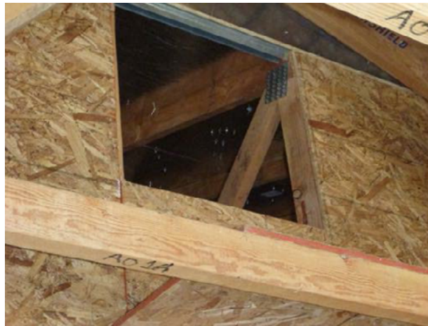
Figure 3-6. Attic access in garage – not penetrating ceiling insulation
