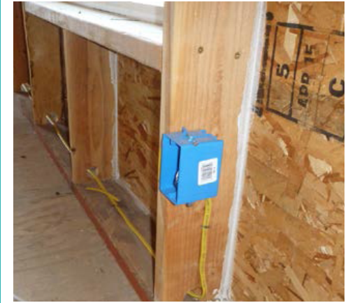
Figure 3-12. Studs pre-drilled for wiring
