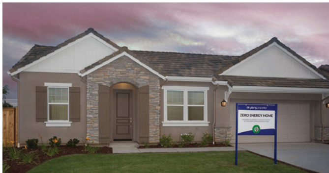
Residence 210i Zero Energy Home at Sierra Crossing, Clovis, CA Michael Rupard, De Young Properties, 2017 Brett Nelson photo
