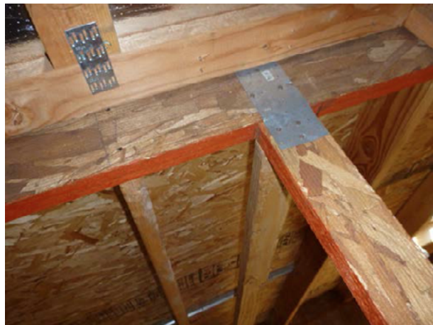
Figure 3-7. Engineered single top plate, from above
