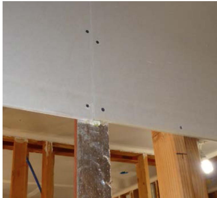
Figure 3-11. Drywall splicing
